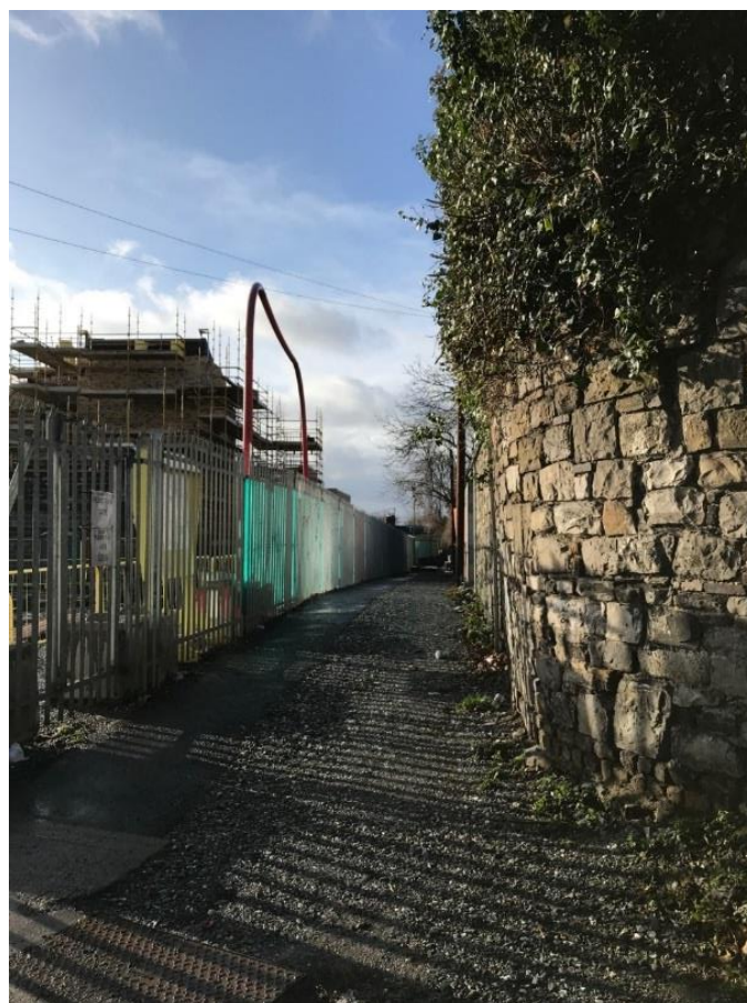
Plate 3.18 Laneway to the rear of No.'s 20-42 North Circular Road. The DCC development is visible on the left.
