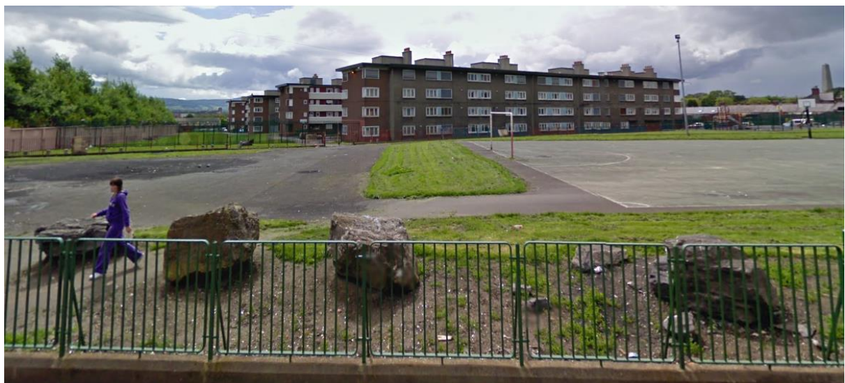
Plate 3.15 Former O'Devaney Gardens Flat Complex (Source Google Maps – Image Captured May 2009)
