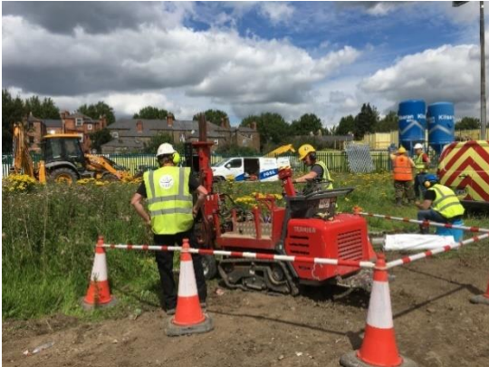
Plate 3 window sampling 'the Dando terrier'
