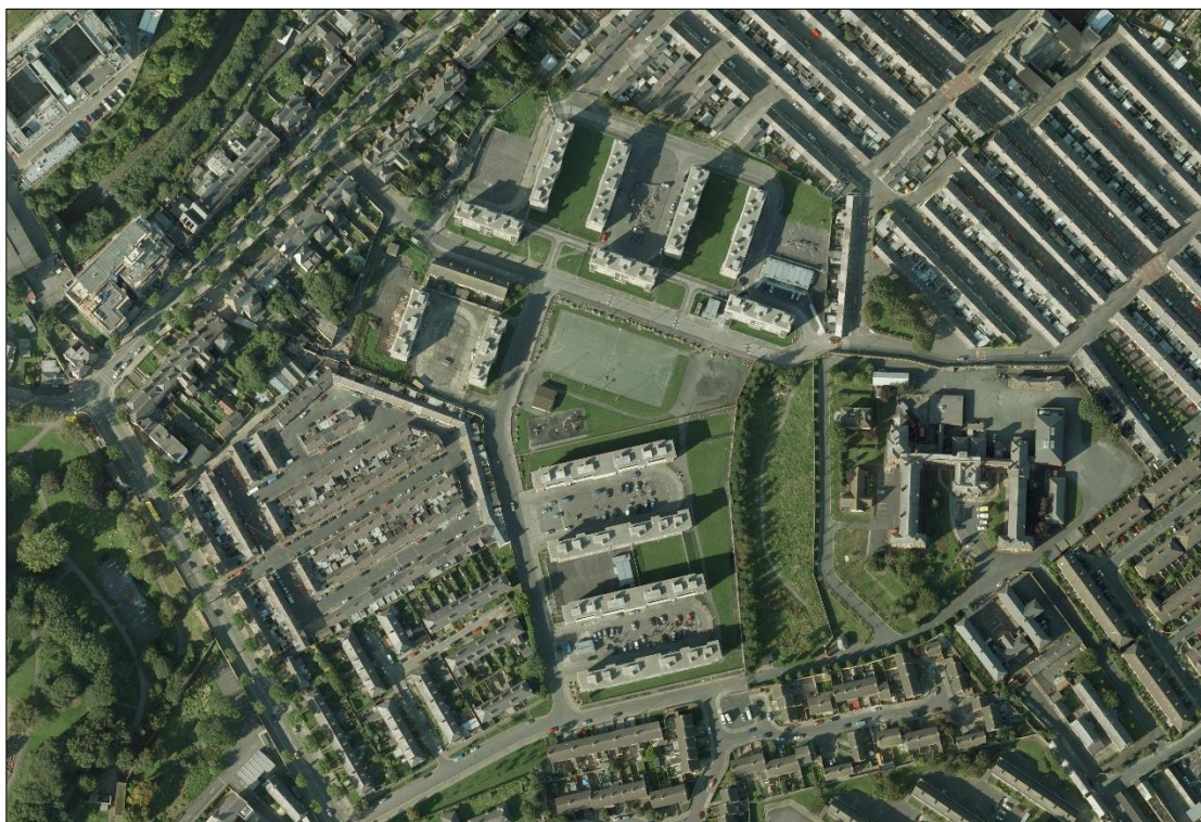
Figure 14.2: O'Devaney Gardens flat complex prior to demolition (2008)
