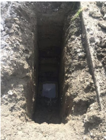
Pate 27 Trench no 26
