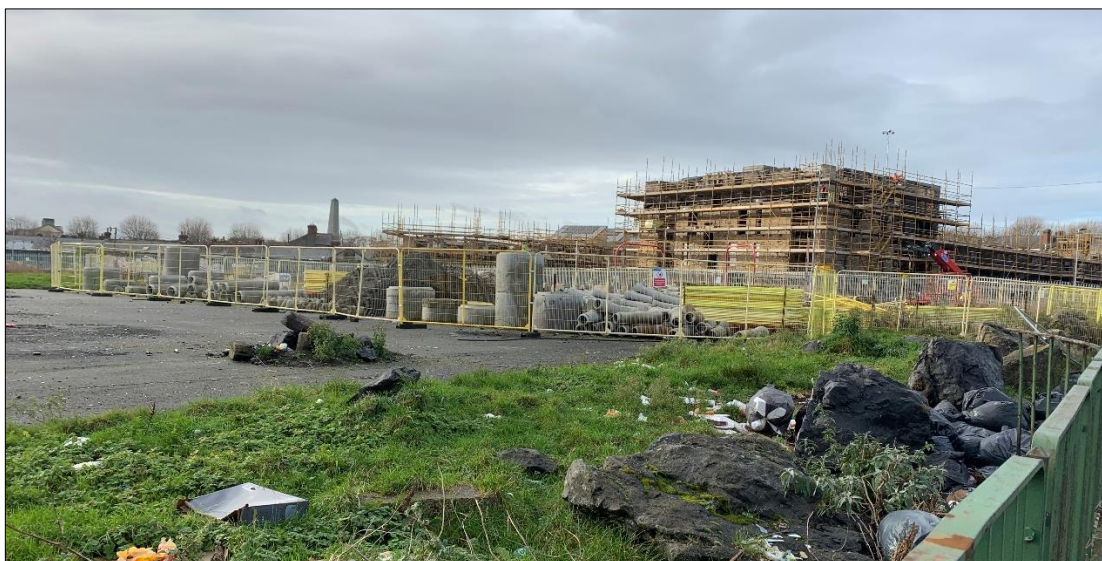
Plate 14.1: Phase 1A under construction near the former O'Devaney Gardens central open space (December 2020)
