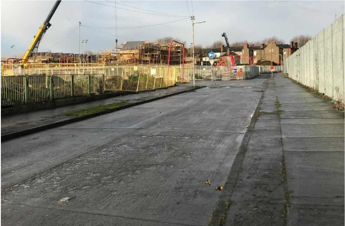
Plate 3.7: Internal road between North Circular Road and Thor Place. The development underway is the DCC Phase 1A development, with part of the current application site in use as site compounds.
