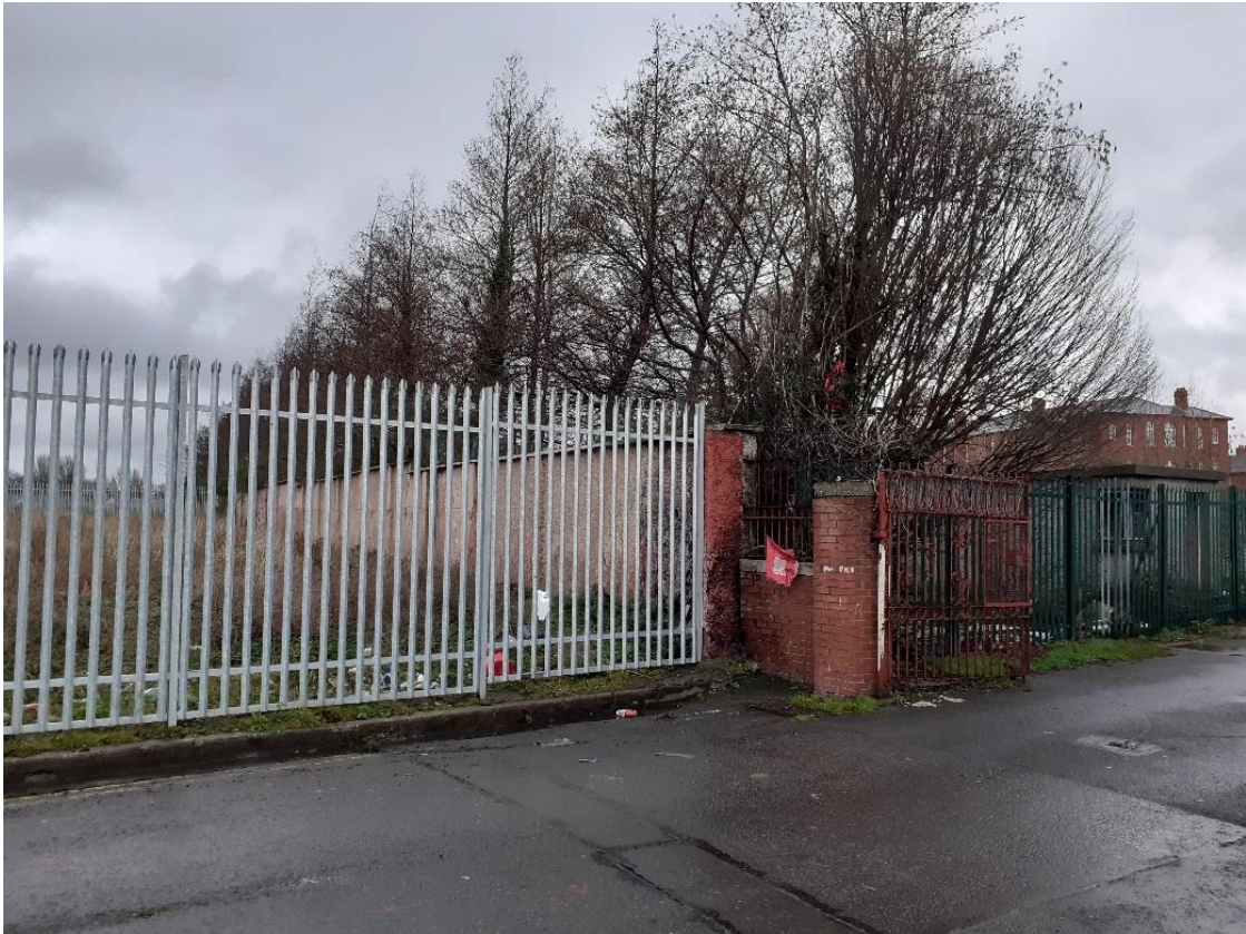
Plate 3.13 Boundary wall between the former O'Devaney Gardens Site and strip of lands formerly part of St. Bricin's.
