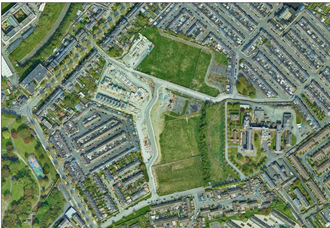
Figure 14.3: The O'Devaney Gardens lands showing Phase 1A under construction (2020)
