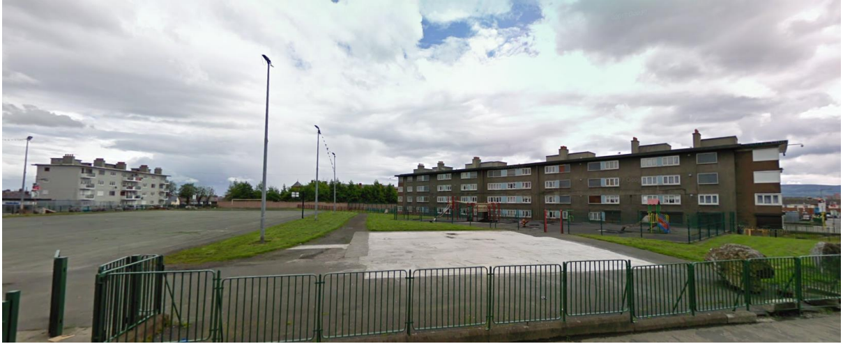
Plate 3.16 Former O'Devaney Gardens Flat Complex (Source Google Maps – Image Captured May 2009)
