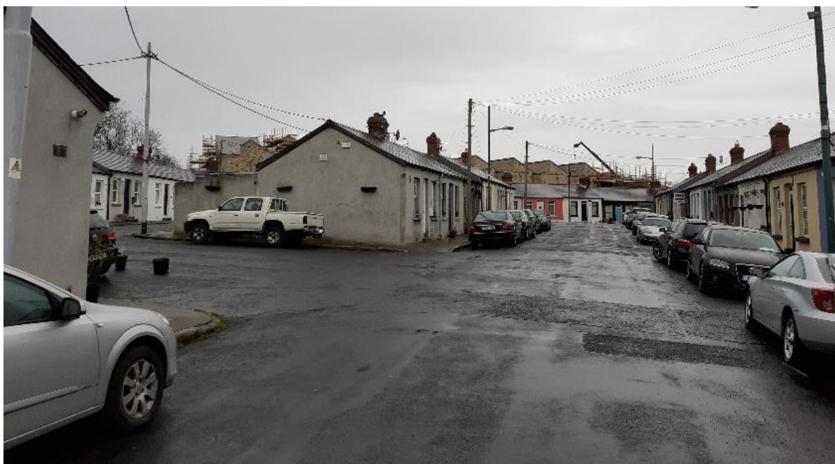
Plate 3.20 Black Street with the DCC development (Phase 1A) visible in the background, behind the cottages on Findlater Street.
