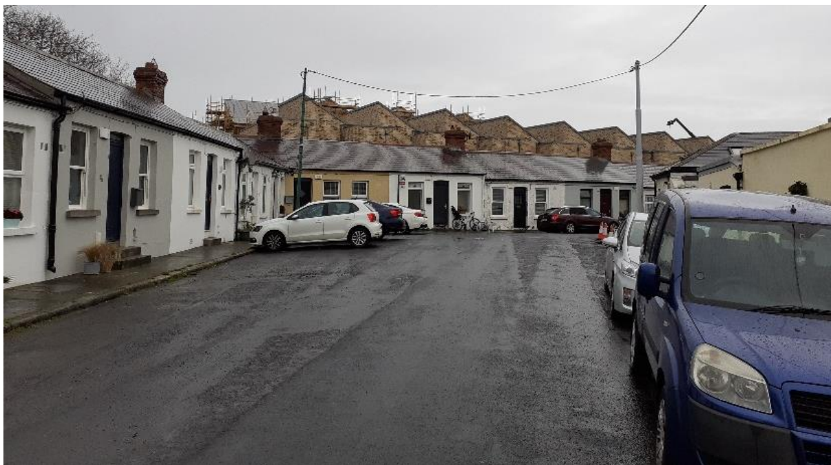
Plate 3.19 Findlater Street with the DCC development (Phase 1A) visible behind the cottages.
