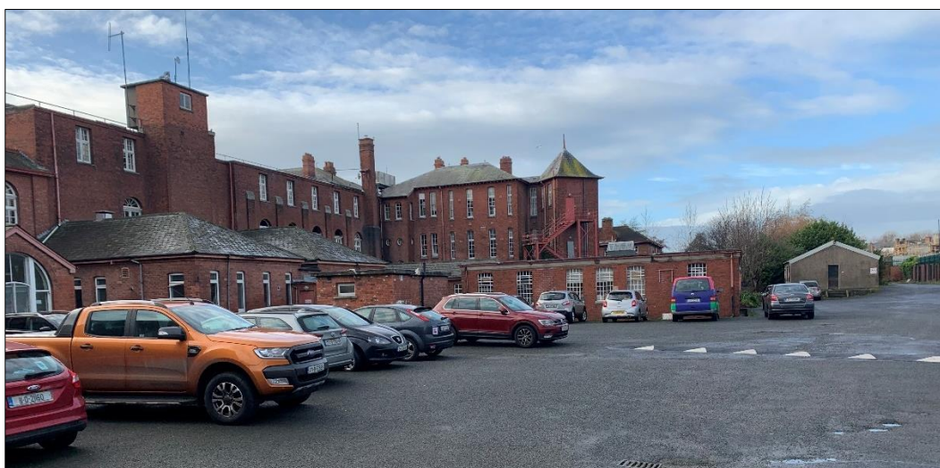
Plate 14.14: A view towards the site from the yard to the north of the main St Bricin's hospital complex
