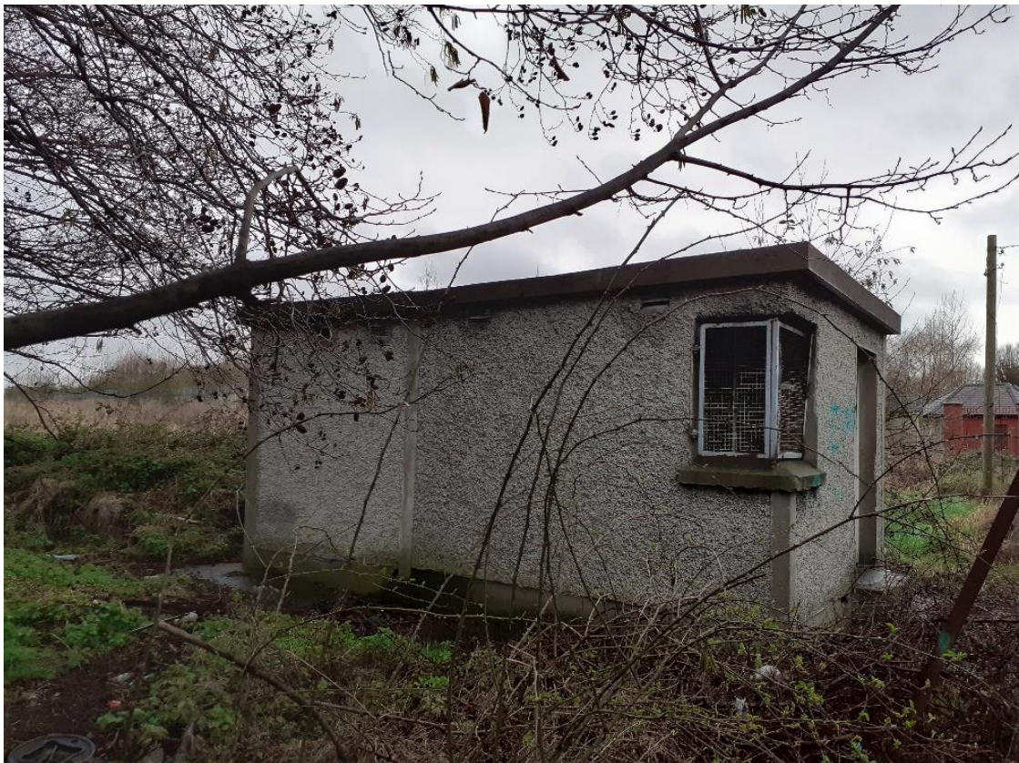
Plate 3.14 Existing building on site (to be demolished)
