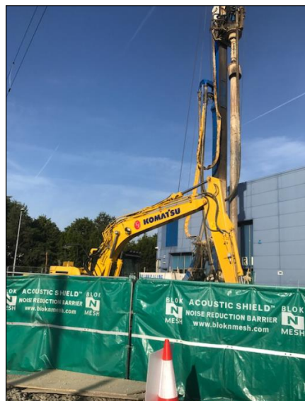
Acoustic blankets screening piling and excavations
