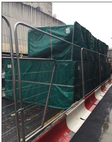
Double height acoustic blanket enclosure
